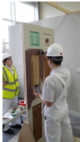
Picture 5 Putting their skills to use on door finishes.
